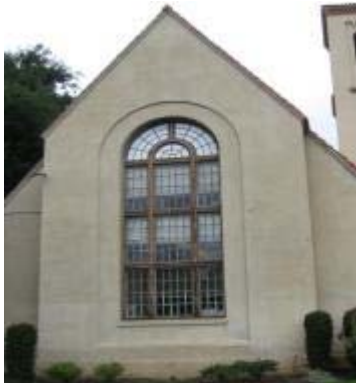
New Tower Bldg. Windows - Before
