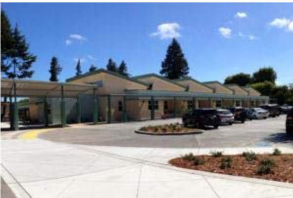
New Classroom Bldg.
