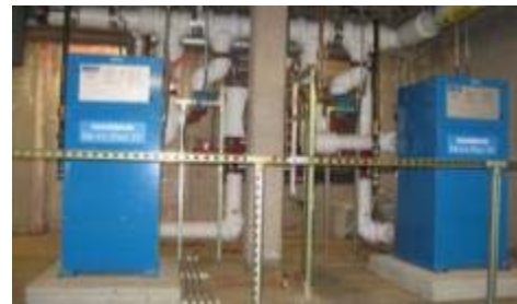
Boiler Replacement - After
