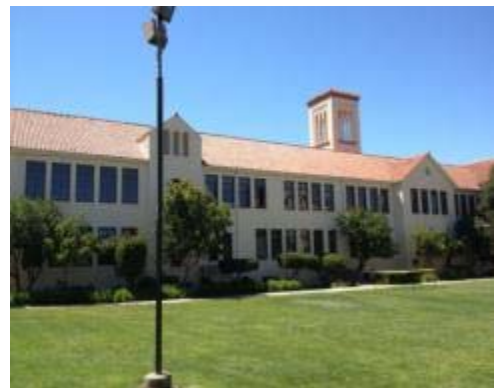
Tower Bldg. New Windows - After
