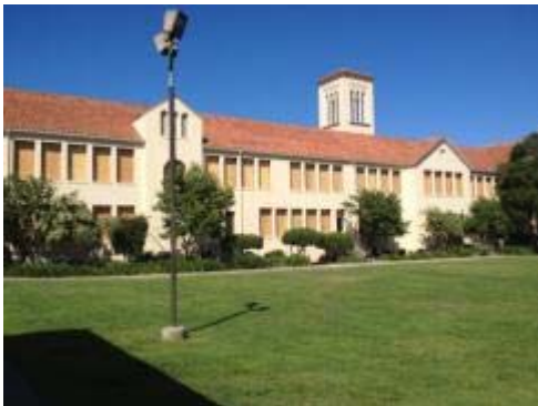
Tower Bldg. New Windows - During
